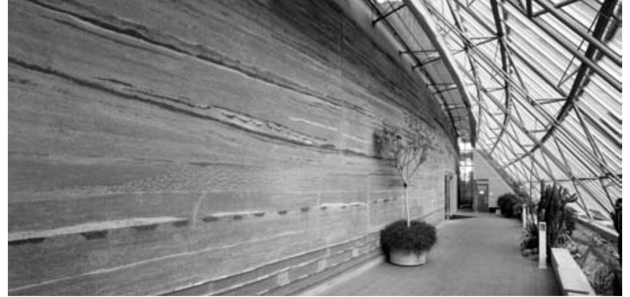
Close-up view of the rammed earth wall at Feldenkirch Hospital, Austria.
