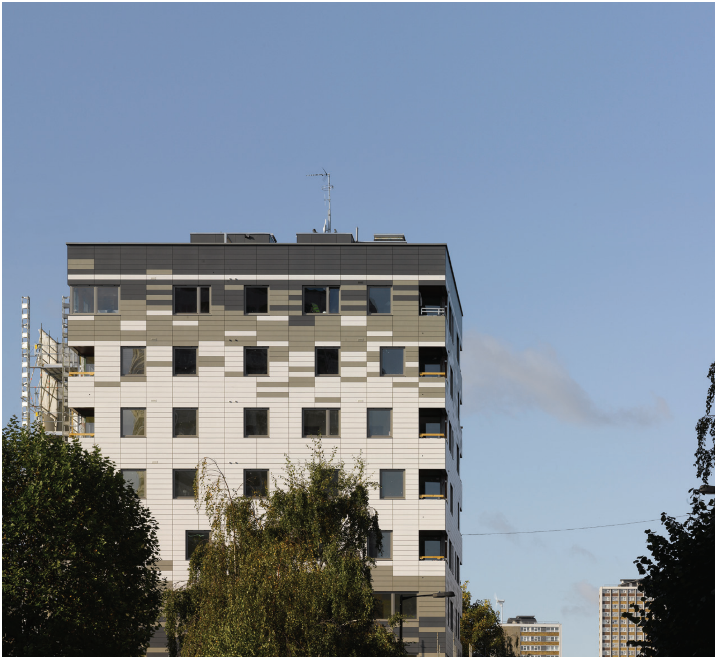
12 Murray Grove in Islington, Waugh Thistleton's first CLT project (2009). This nine-storey building propelled the practice principals into the limelight as international ambassadors for the engineered-timber revolution
