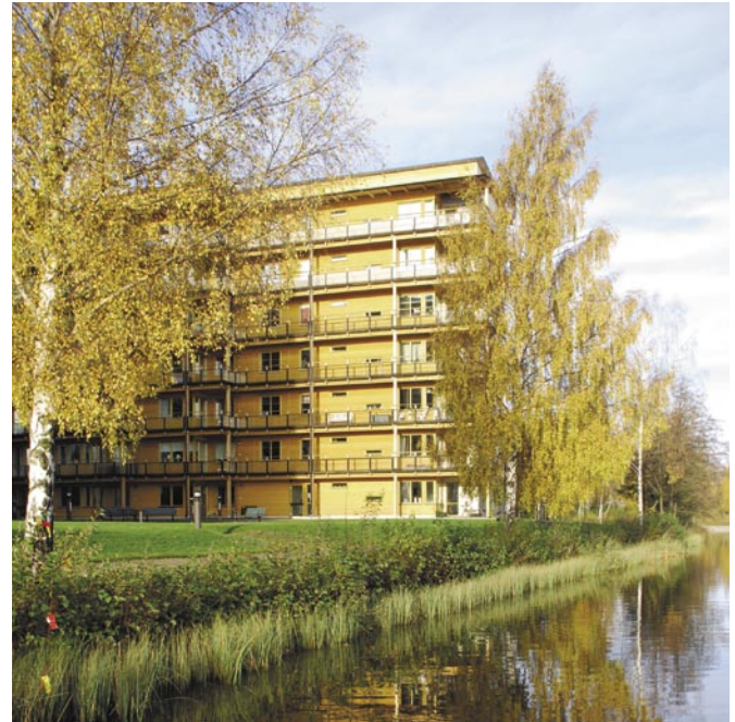
The Swedish town of Vaxjo is an unlikely epicentre of timber hi-rise. Hi-rise may be too vertical a description for eight storey buildings but even so what is happening in Vaxjo remains remarkable, and is a beacon for what can be achieved. In the last year, 4 eight storey cross-laminated apartment blocks have been completed there.
