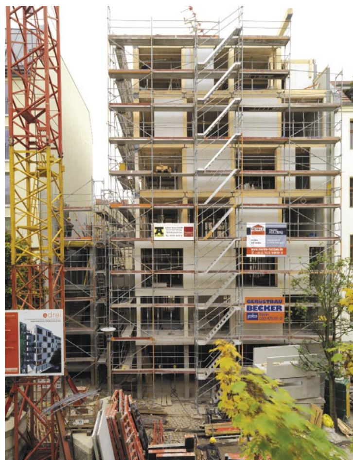
This photo and opposite: ‘E3’, a seven-storey infill apartment block in Berlin seems to have caught the imagination in Germany’s biggest stone-centric city. Although heavily regulated for fire risk, the architects were able to satisfy the city’s planning officers and fire brigade with the timber system.
