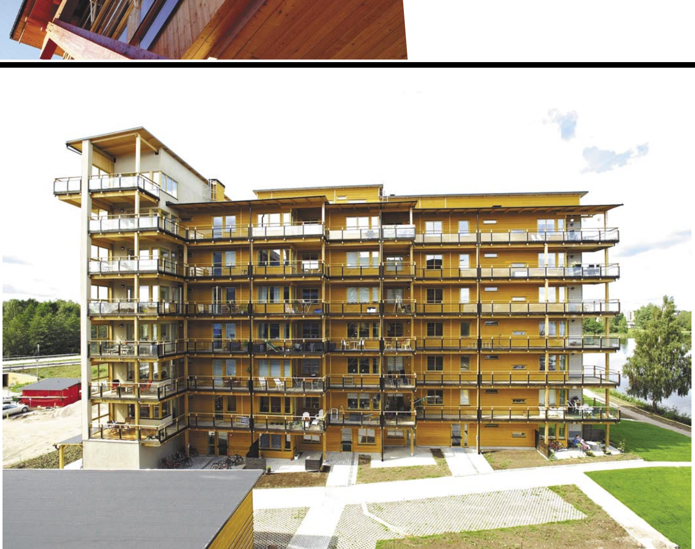
Drawn around a cross between a T and a semi-triangular plan, each of the four cross laminated timber buildings narrow towards the lakeside front. Each floor contains 5 apartments and each block 134 apartments.
