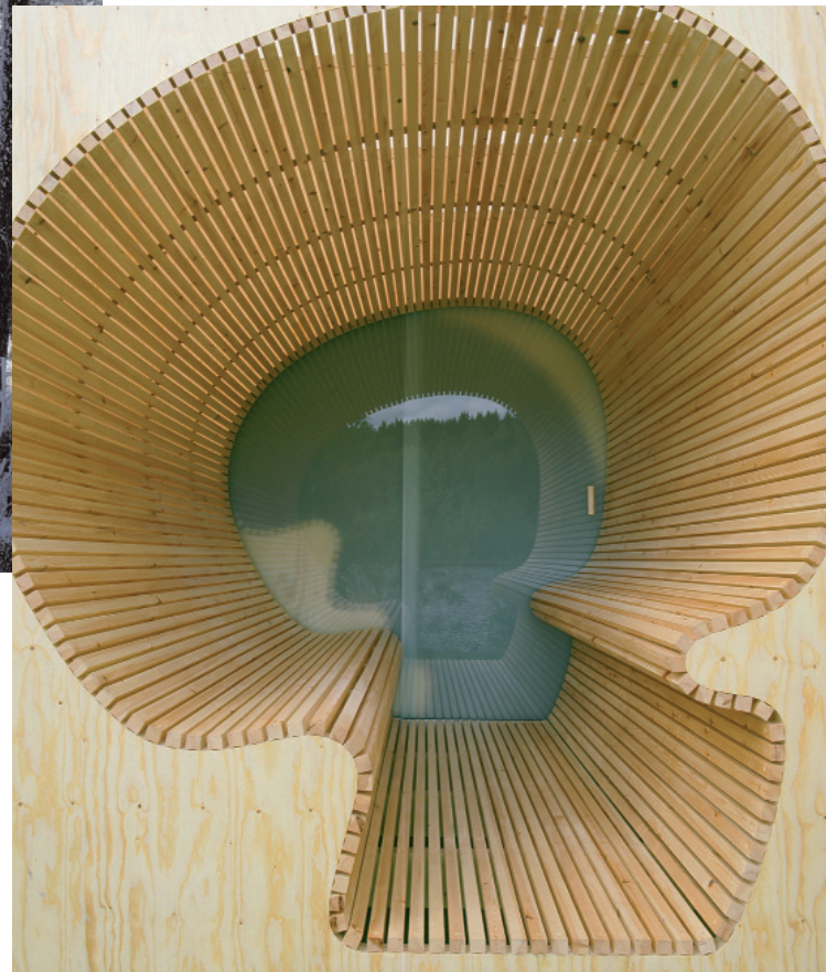
Left: Forest rester 2001/2's Aitta guest house. Several woods, including larch, aspen, spruce, oak and alder, were applied to make the truss and walls.
